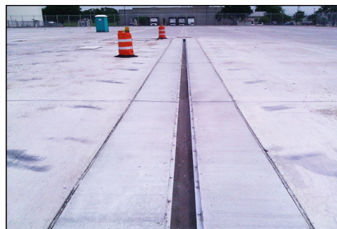
EPS foam forms removed
