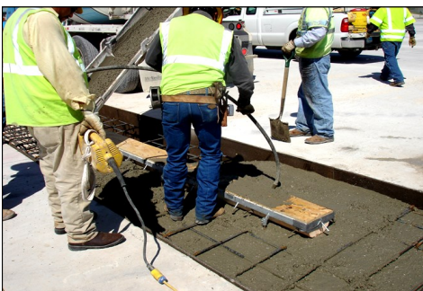
Placing concrete & vibrating
