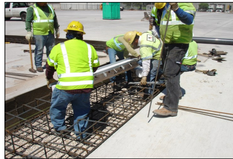
Installing EconoDrain 8' long sections
