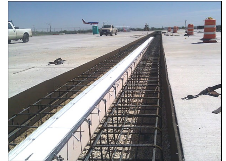
Frames secured with alignment clips
