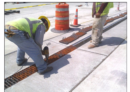
Completed trench drain and grate
