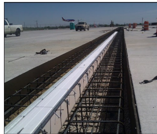
EconoDrain system installed, aligned and leveled with #4 rebar inserted through anchor stands and driven into earth.
