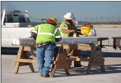
Applying form release to foam forms
