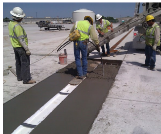
Place concrete per installation instructions and vibrate concrete on each side of EPS forms.
