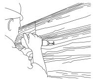
2) Drill Slots Drill or route slots at the intended tie locations. Slots should be 5/16" wide and 7/8" tall to allow the loop to comfortably slide through.
