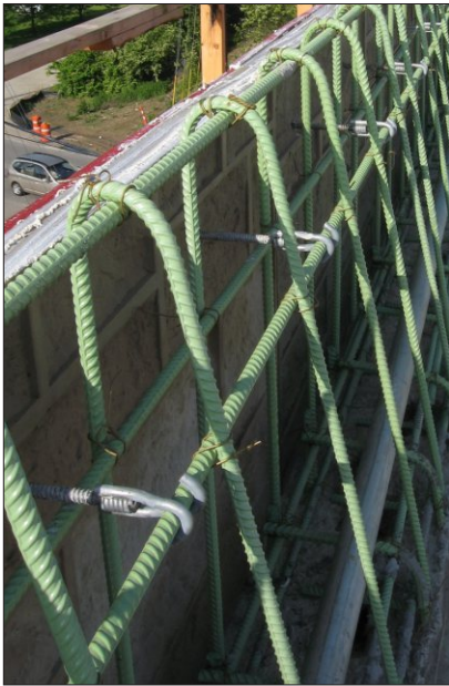
Attachment of plywood-backed form liners for slip-formed highway barriers. Galvanized RH-6.
